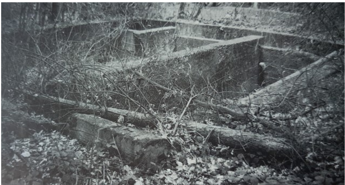
Figure 39 The remains of the concrete sewage plant. (Fareham, Clipstone Camp an account of a military training camp of the First World War , 1994, p. 10)
