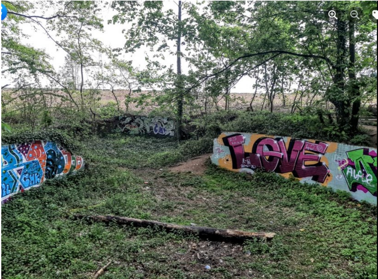
Figure 42 The Sewage filter Beds (Priestley, WW1 Clipstone Camp, 2020)
