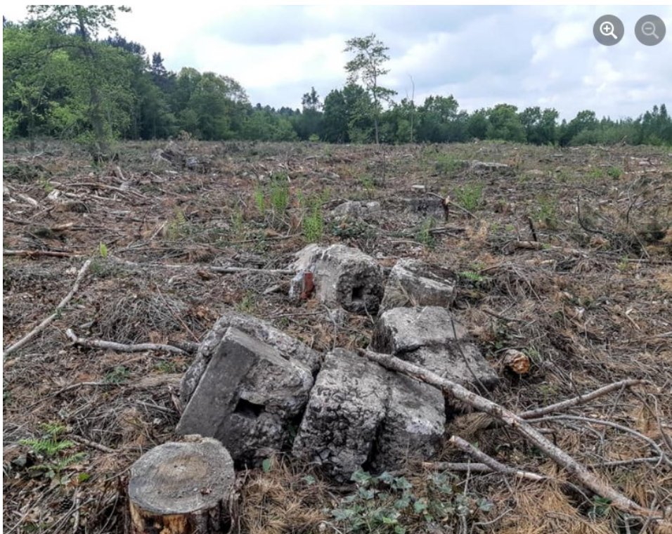
Figure 76 Hospital Site Clearance 2 (Priestley, WW1 Clipstone Camp, 2020)
