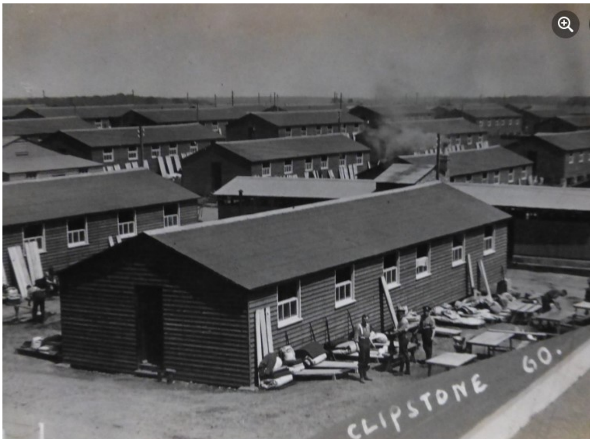
Figure 6 Barrack huts with bedding and tables outside (Historic photo ref 13).
