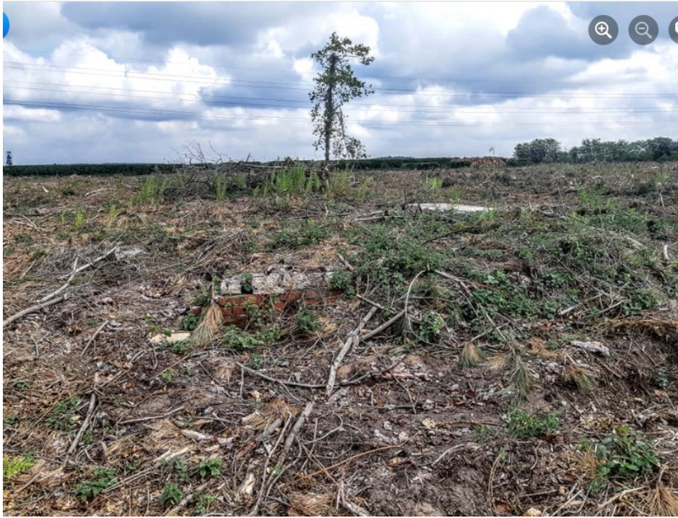
Figure 83 Hospital Site Clearance 9 (Priestley, WW1 Clipstone Camp, 2020)
