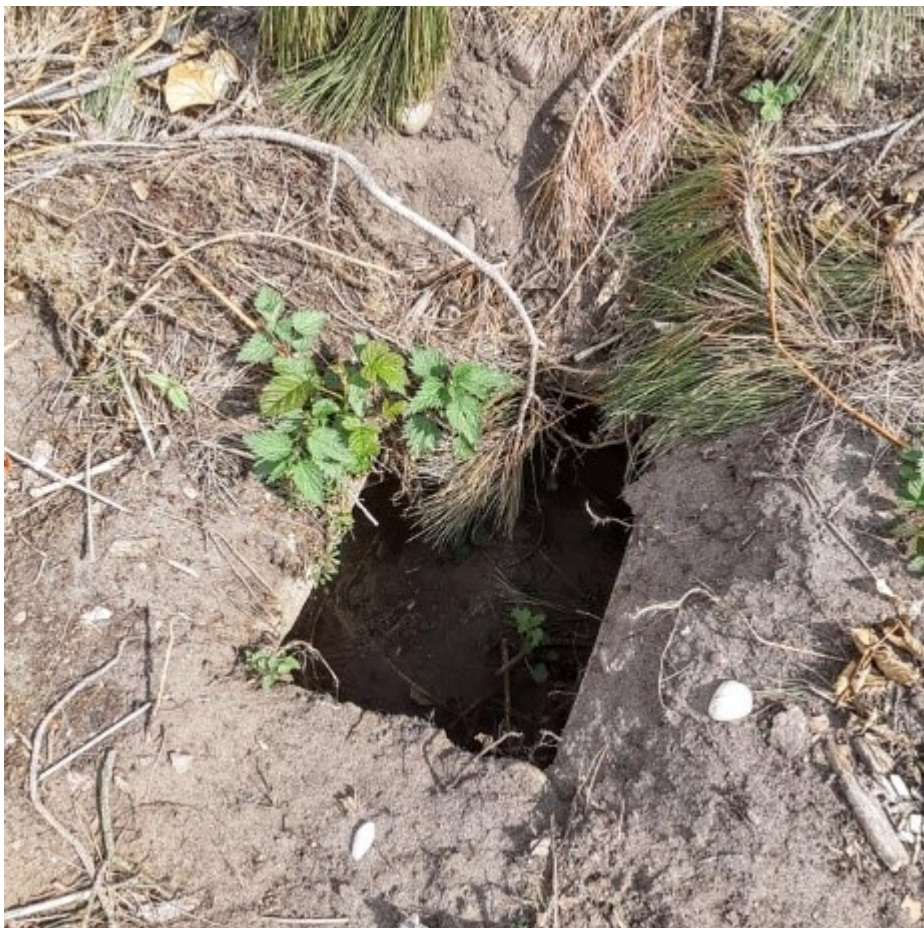
Figure 80 Hospital Site Clearance 6 (Priestley, WW1 Clipstone Camp, 2020)
